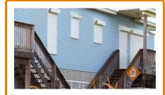
Storm shutters are used to prevent windows from breaking during disasters like a hurricane. It's a simple solution to prevent a lot of damage. Flying debris can break windows or even hurt people inside.
