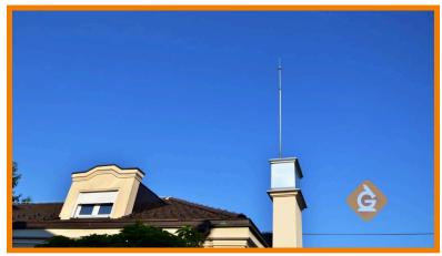
lightning, but we can direct its energy into the ground to prevent an electrical surge, which can damage electronics. Lightning rods are made of metal and used to transfer the energy of a lightning bolt to the ground through wires. This directs the electricity through the rod and then straight to the ground, instead of through the building.
